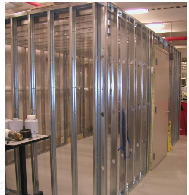
Fumigant Demonstration Chamber Public Health Agency of Canada
